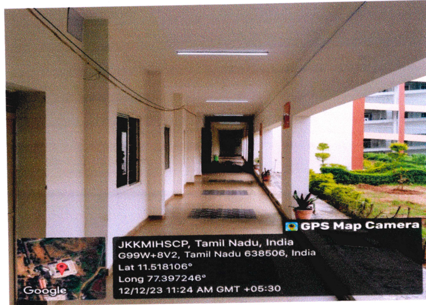
PHOTO OF LED BULBS IN MAIN BUILDING
