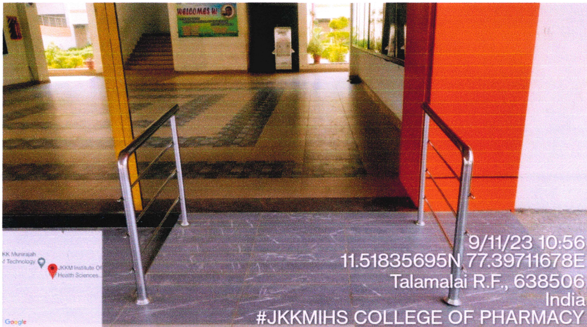
PHOTOS OF RAMP IN MAIN BUILDING ENTRANCE ON 09.11.2023
